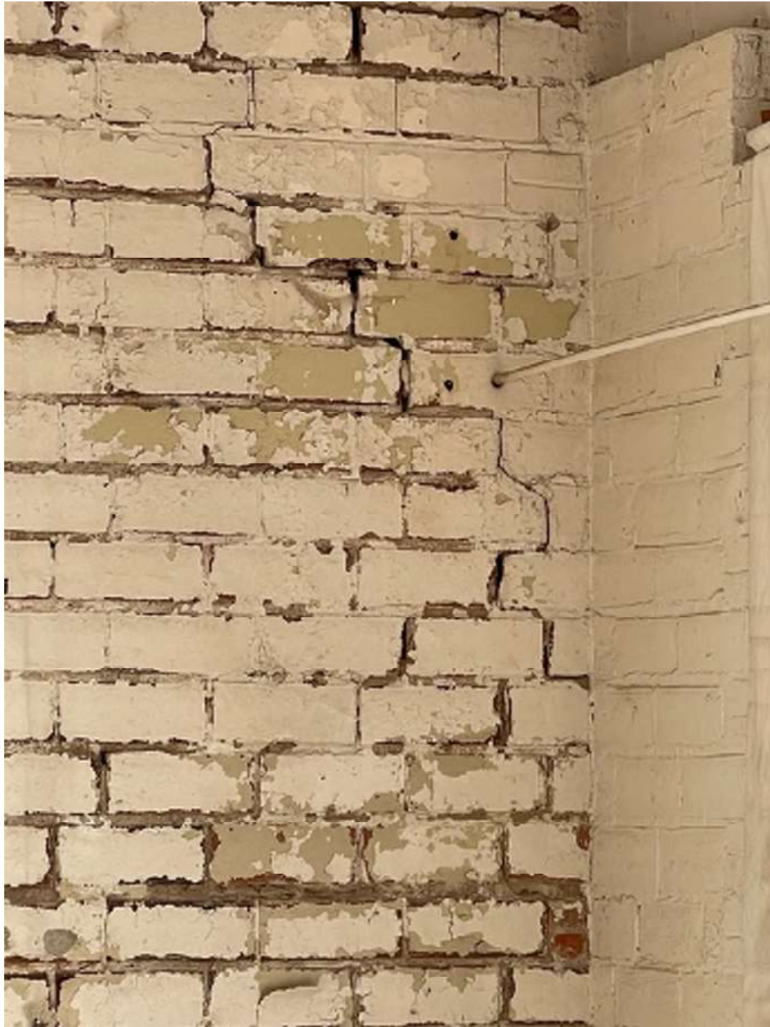
Photo 16 - Vertical stair stepped crack at Southwest corner due to settlement
