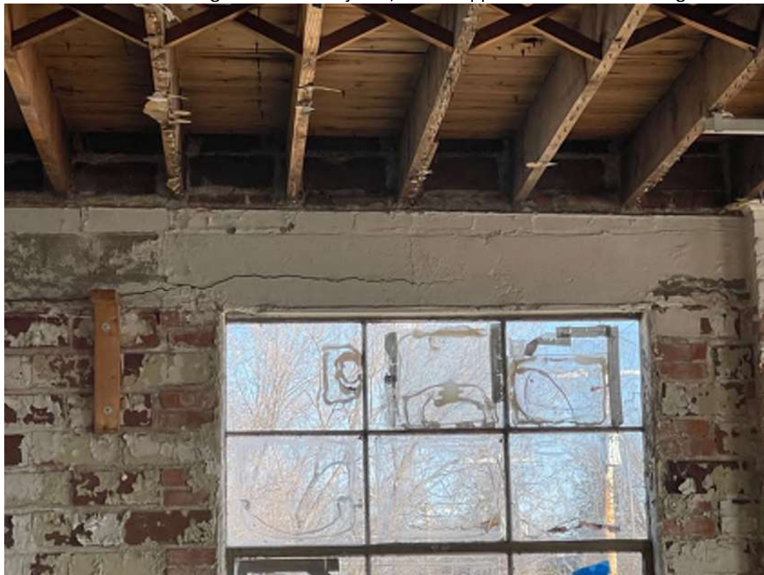
Photo 22 - Roof 2x10 joist nearing on cracked concrete beams and lintels over the windows
