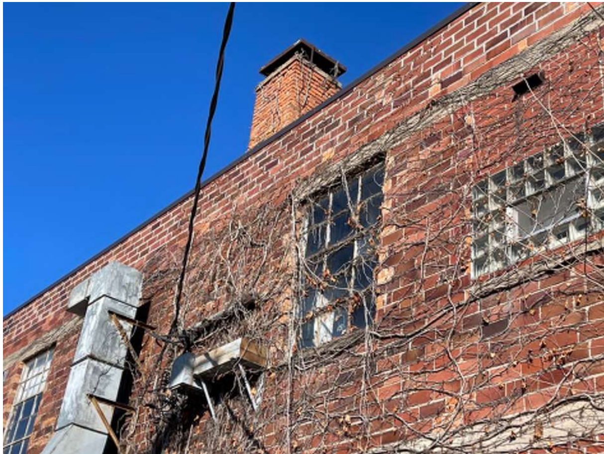
Photo 7 – East half of the South side exterior wall is covered with vines. Over time vines contribute to the deterioration of the masonry. Recommend killing and removing them.
