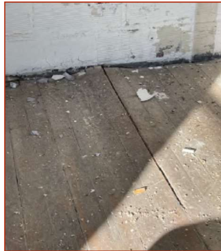
Failing exterior bricks on exterior wall and buckling of hardwood flooring. Source: Select Structural
