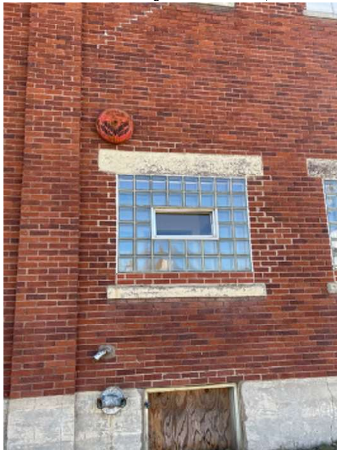
Photo 13 – Front brick facade with previous repairs to brick and mortar joints
