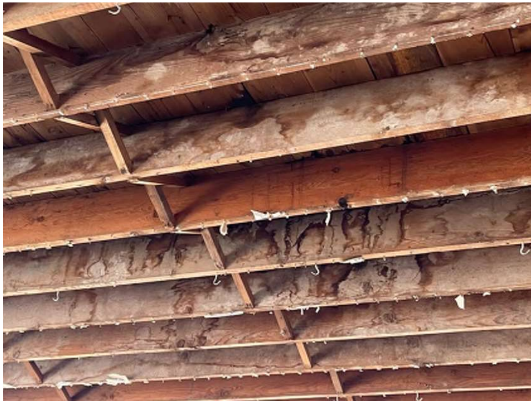
Photo 21 - Water staining found on roof joists, but no apparent structural damage from rot
