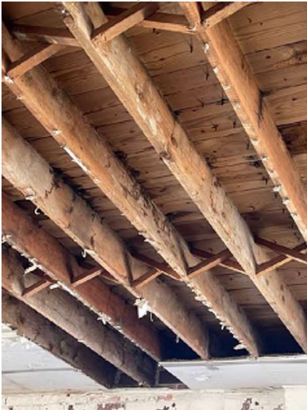
Photo 20 - 2x10 Roof joists @ 16"o.c. with x-bridging. Light water staining, but in good condition
