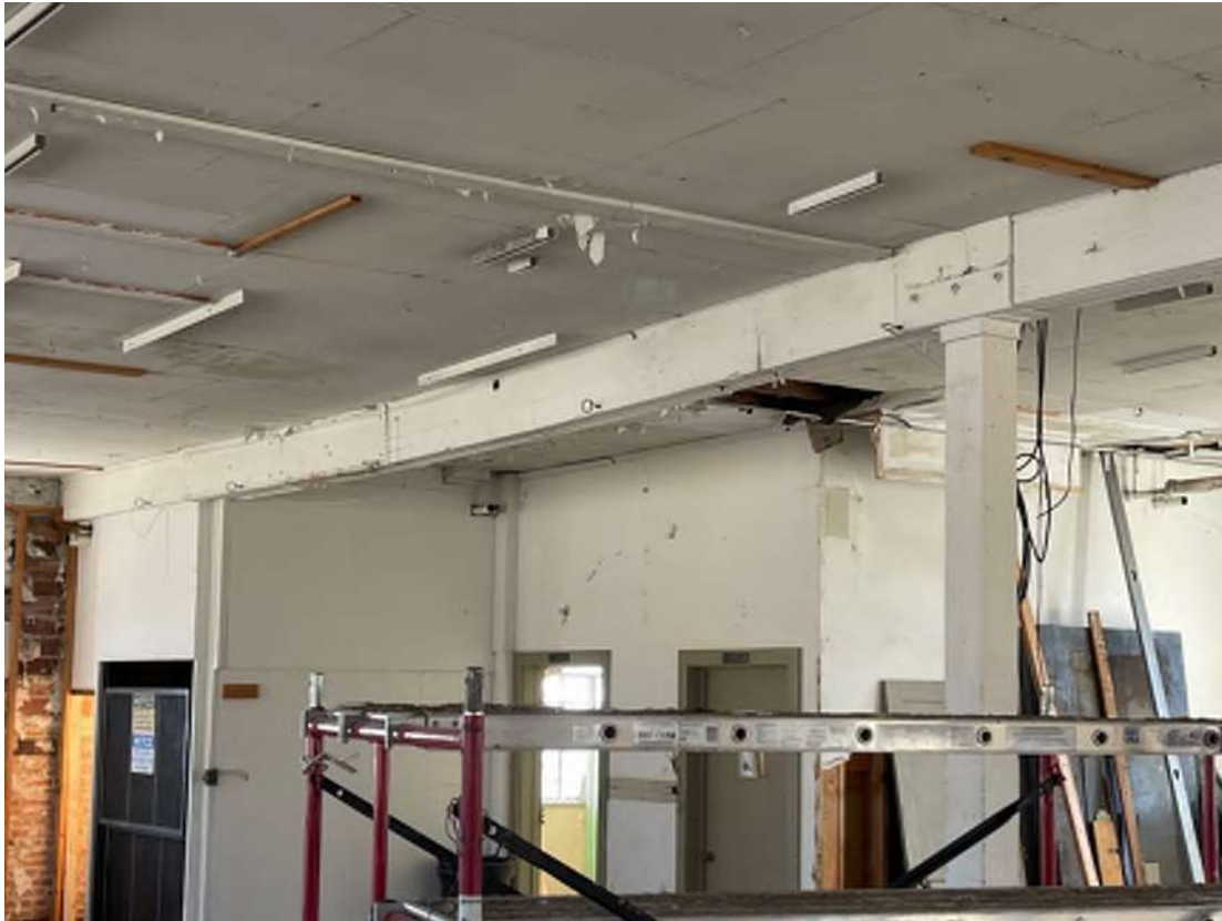
Photo 28 - Sagging beam found at the East end supporting the roof near the elevator shaft. Evidence of former mechanical equipment hung from the ceiling in this area may have overloaded the beam, coupled with water from roof leak may have caused this sag. Jack back into place and nail 2x to each side of the beam as reinforcement.
