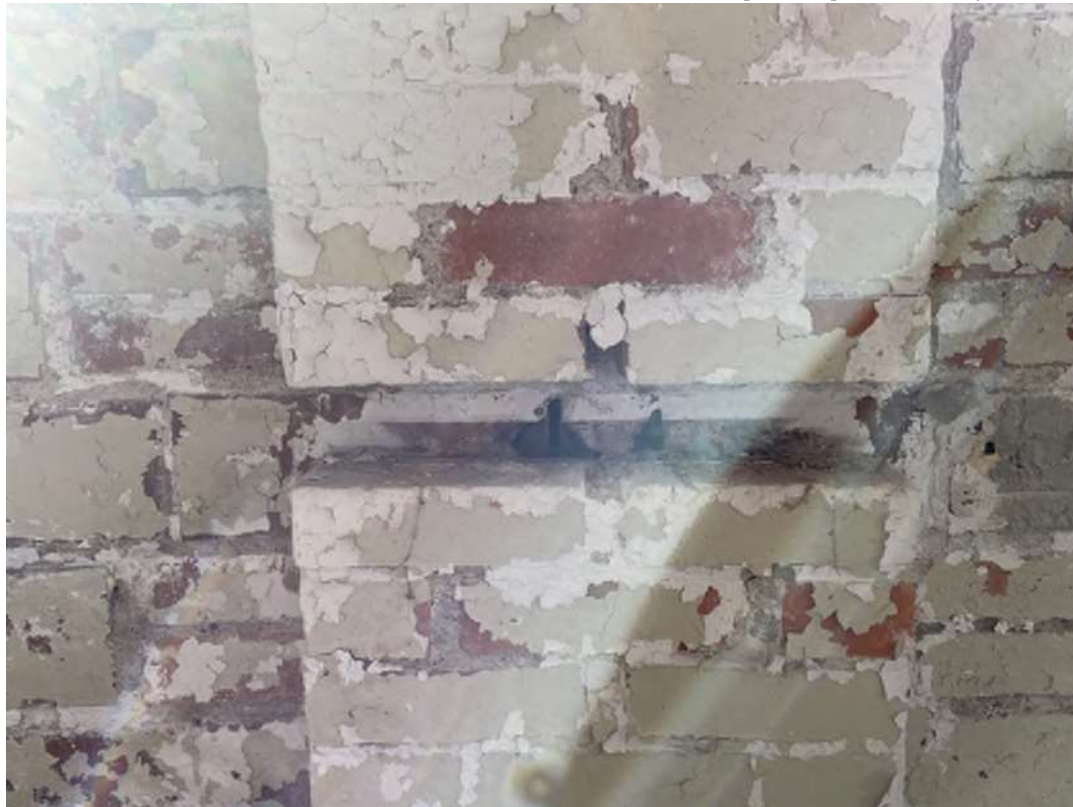
Photo 18 – Bricks removed from pilaster/pier likely to install electrical conduit. Recommend replace
