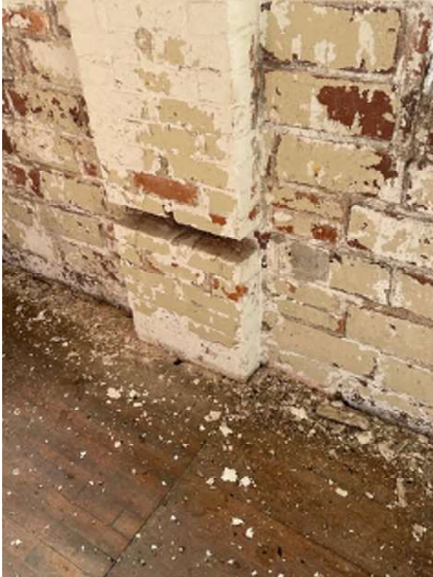
Photo 19 – Additional gap in missing brick pilaster
