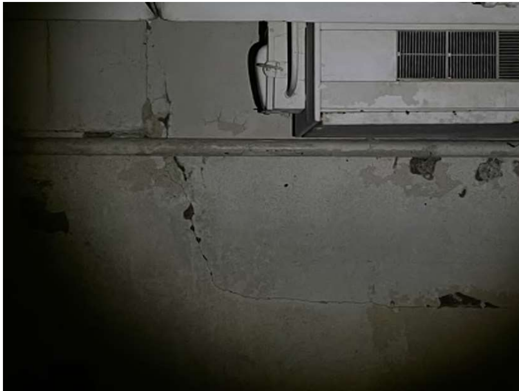
Photo 32 - Cracking of foundation wall in basement Northside wall
