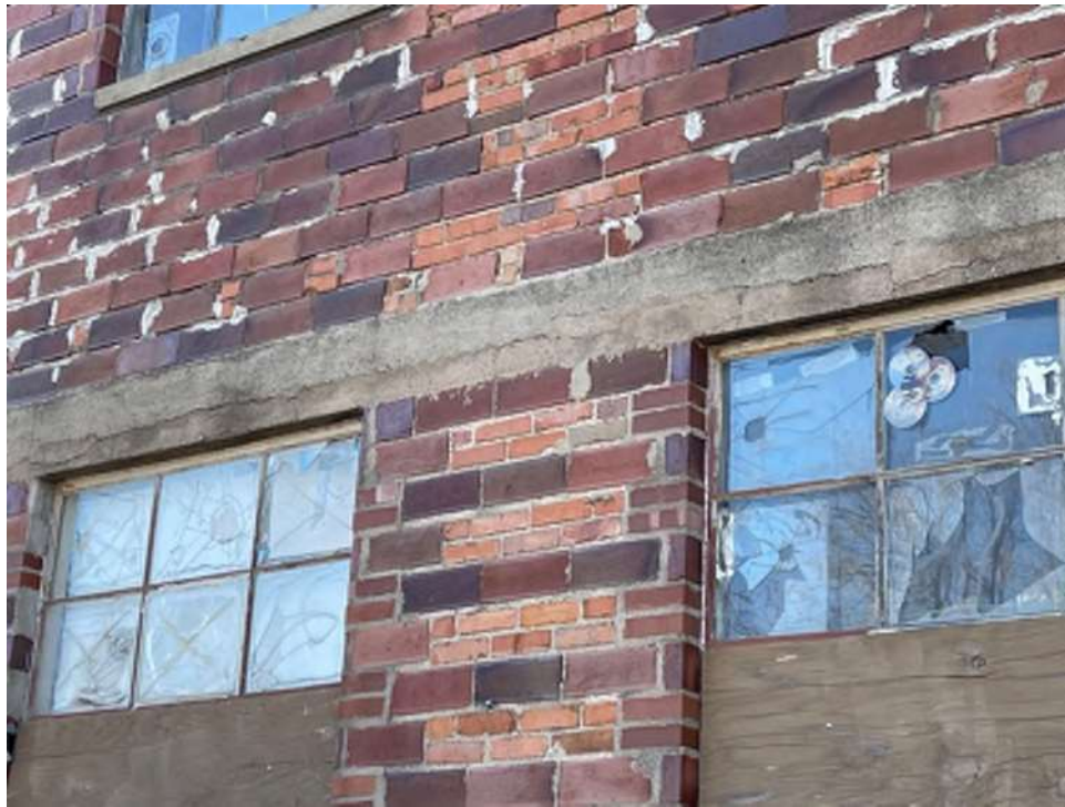
Photo 12 - Lateral cracking in concrete beam/lintel. Eventually will worsen and concrete will fall away
