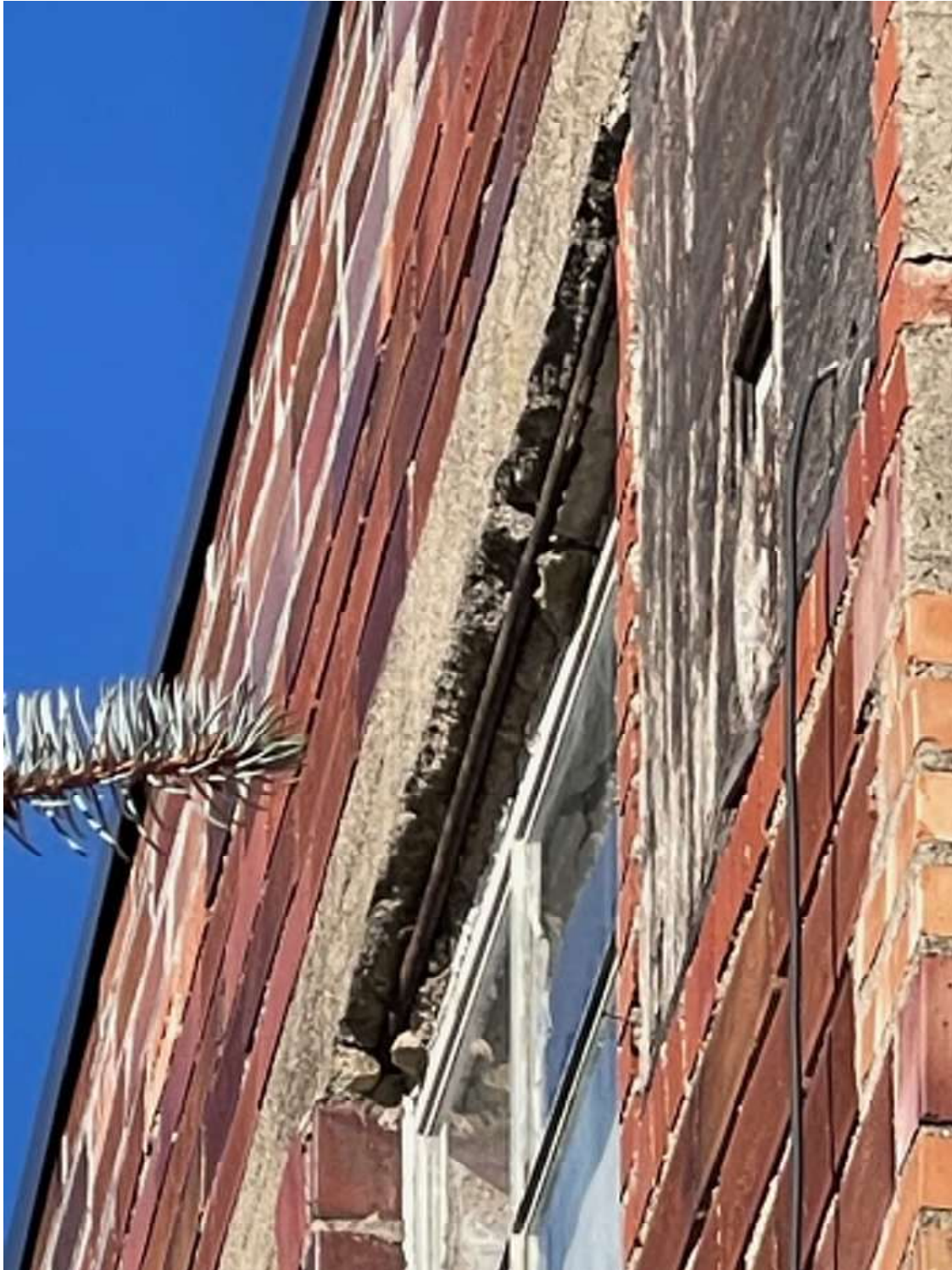
Photo 8 - Exposed structural rebar in concrete lintels that act as beams to carry the roof above the windows. Concrete has broken and fallen away. Recommend lintels be repaired and replaced as needed by the mason.
