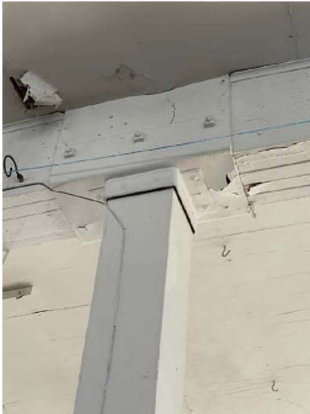
Photo 27 - Steel bracket and saddle found at the beam to column connections. Good condition
