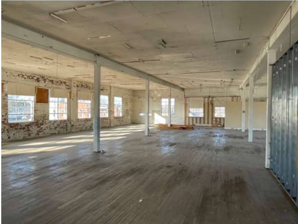
Photo 26 - Overall view of second floor ceiling looking West with column and beam lines running down the center of the building. Much of the ceiling/roof structure in this area was covered with paneling.
