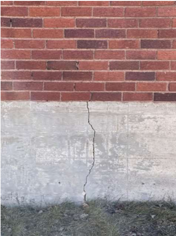
Photo 35 - Vertical cracking at front of building
