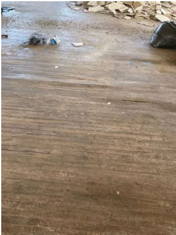
Photo 25 - Minor warping and buckling in wood floor boards due to previous roof leaks
