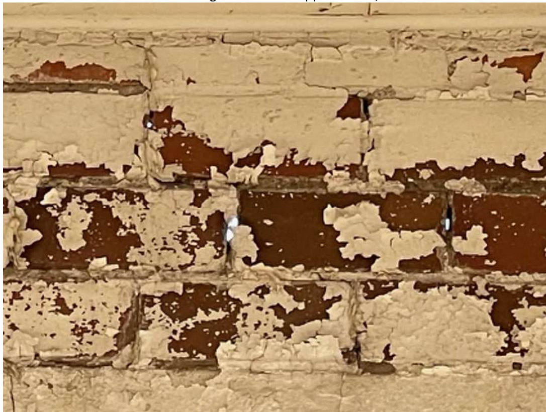
Photo 15 - Mortar deterioration, and gaps in brick showing daylight
