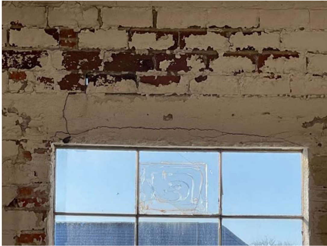
Photo 14 – Interior view of cracking at concrete support beam/lintel
