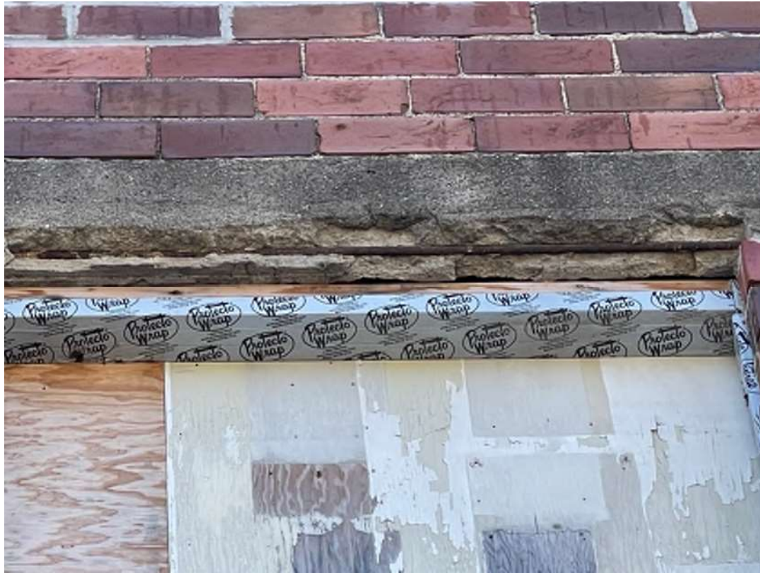
Photo 10 - Exposed rebar and falling concrete support beam/lintel
