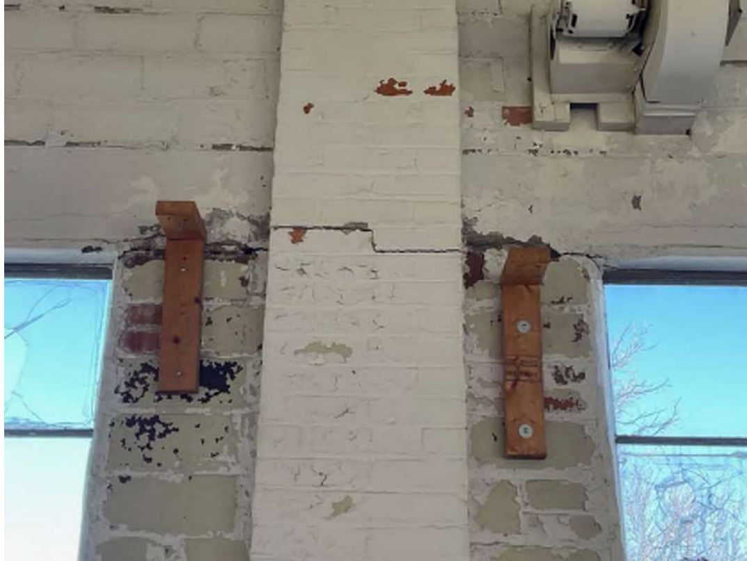
Photo 17 - Crack at concrete beam/lintel on outside is showing through the brick pilaster on the inside
