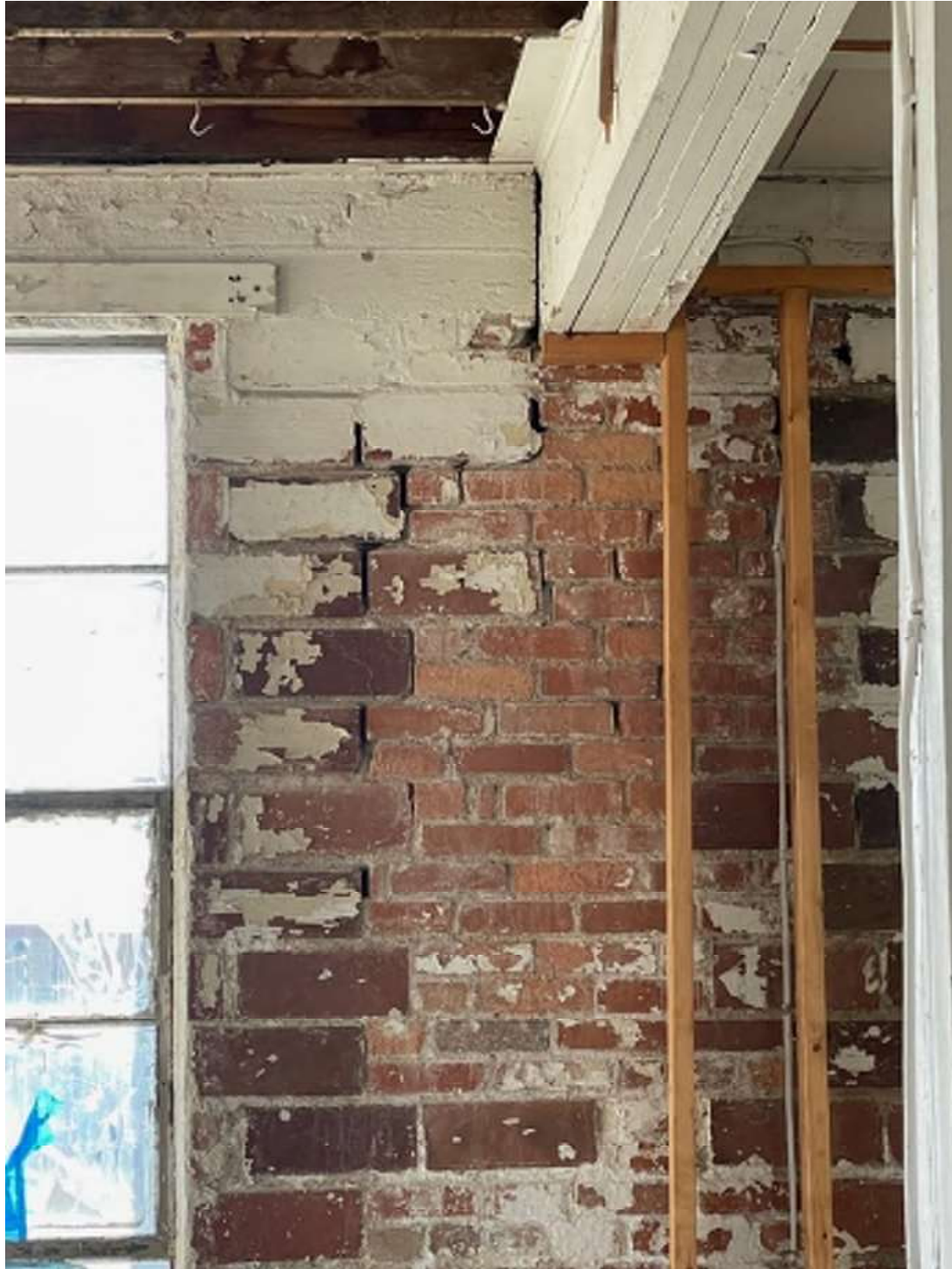
Photo 29 - Roof beam pocketed into masonry wall. Loose bricks need repaired.
