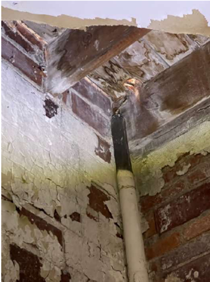
Photo 23 - Second floor 2x12 joist bearing on masonry exterior walls
