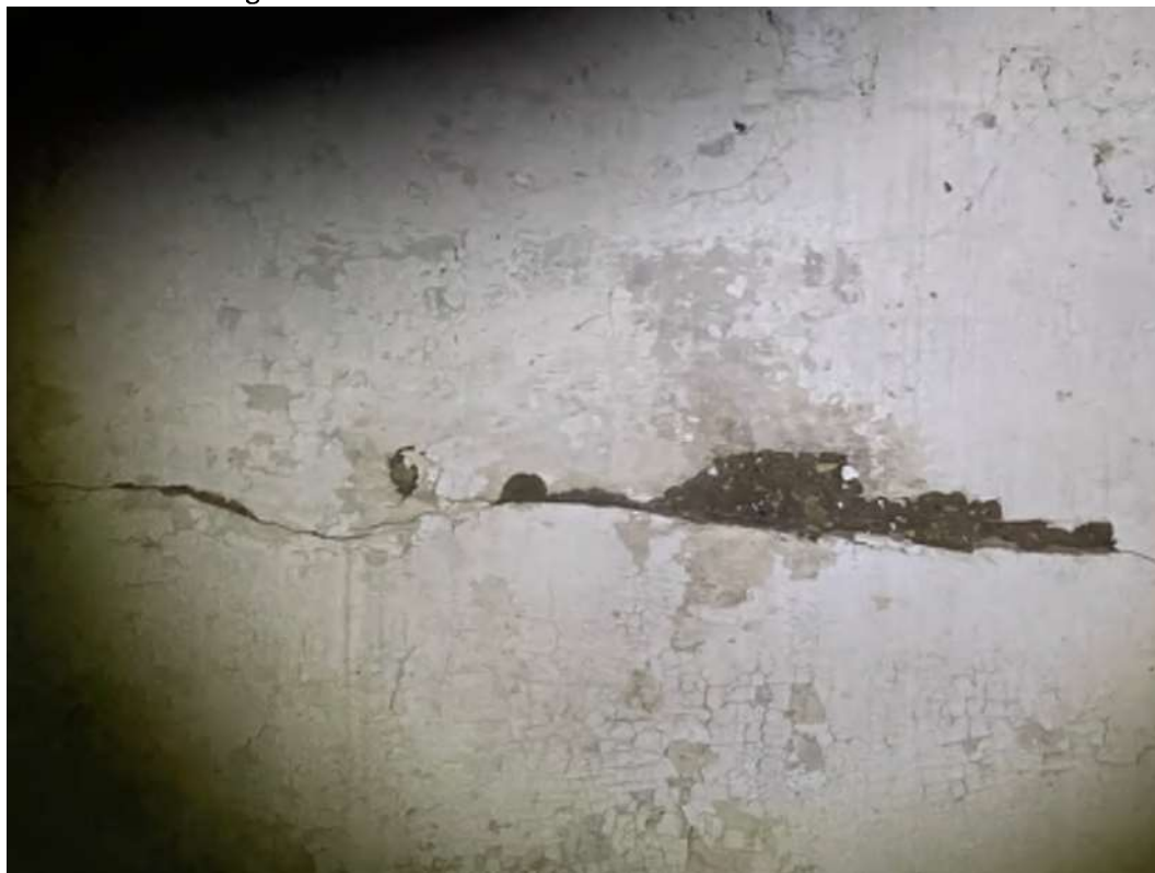
Photo 33 - Cracking of foundation wall in basement Northside wall
