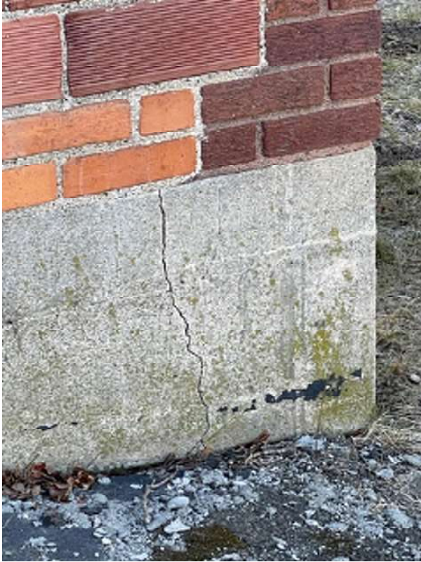
Photo 34 - Vertical settlement crack at building corner
