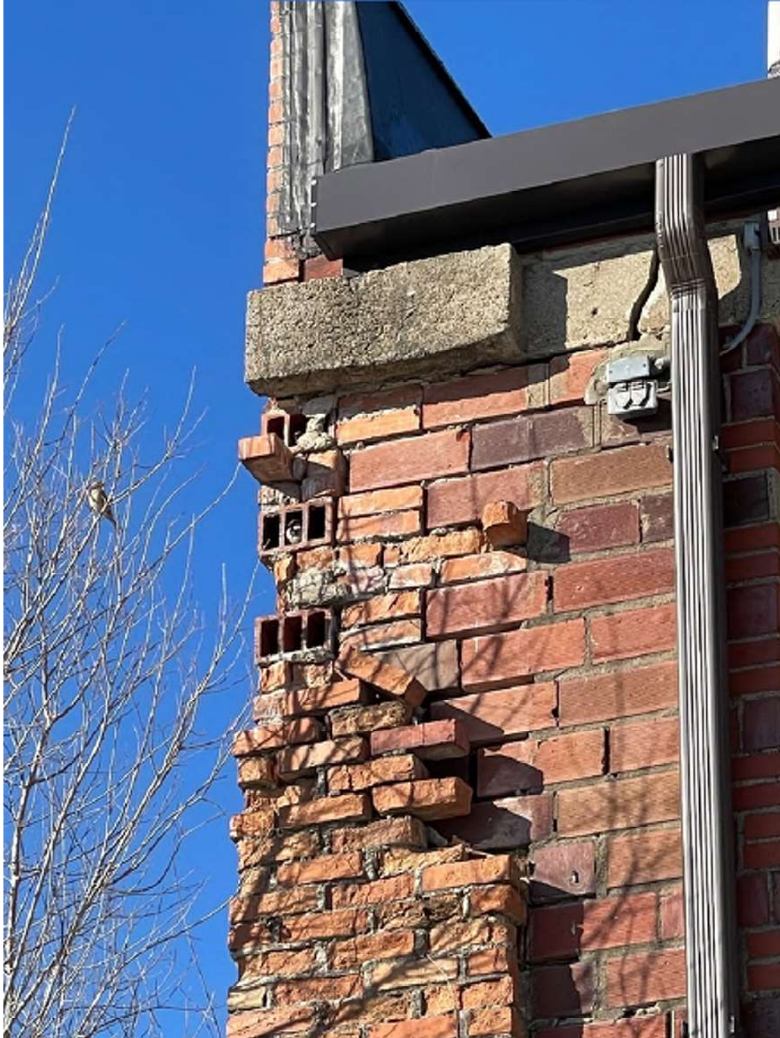
Photo 6 - Falling exterior bricks at Southeast corner of exterior wall. Recommend repairing and replacing as a part of the overall tuckpointing and masonry restoration operations.
