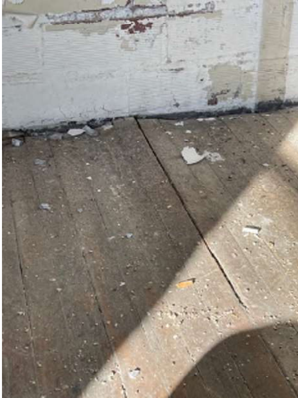
Photo 24 - Buckling of hardwood flooring due to previous roof leak. Structure not visible for review. Hardwood floor covering non-structural.
