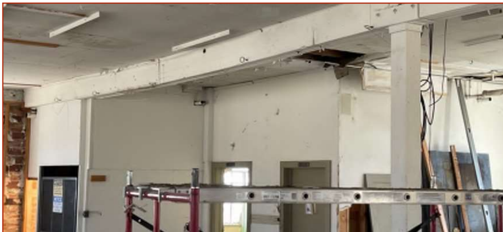
Sagging beam supporting roof near the elevator shaft. Source: Select Structural
