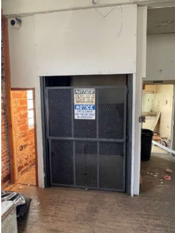
Photo 1 - Freight Elevator Located in Southeast Corner. Was not operable at time of inspection and the structure was covered with limited areas to see. Consult with an elevator company about the possibility of re-using this.
