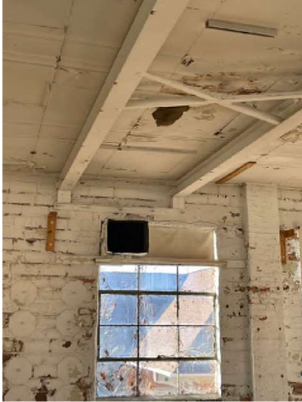
Photo 30 - Steel beam framing from apparent previous machinery support
