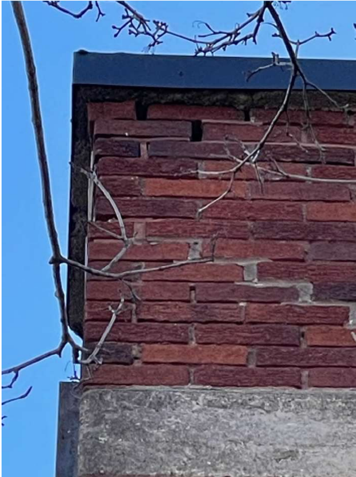
Photo 5 - Loose bricks found at top corner of exterior wall. Non-structural façade, but should be re-set and mortar repaired during tuckpointing.
