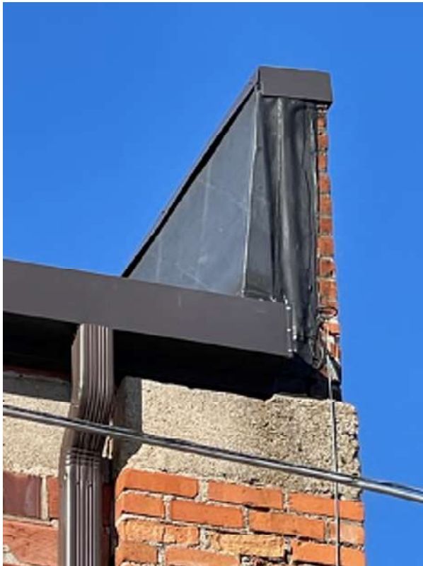
Photo 31 - New roof covering extending up back side of parapet
